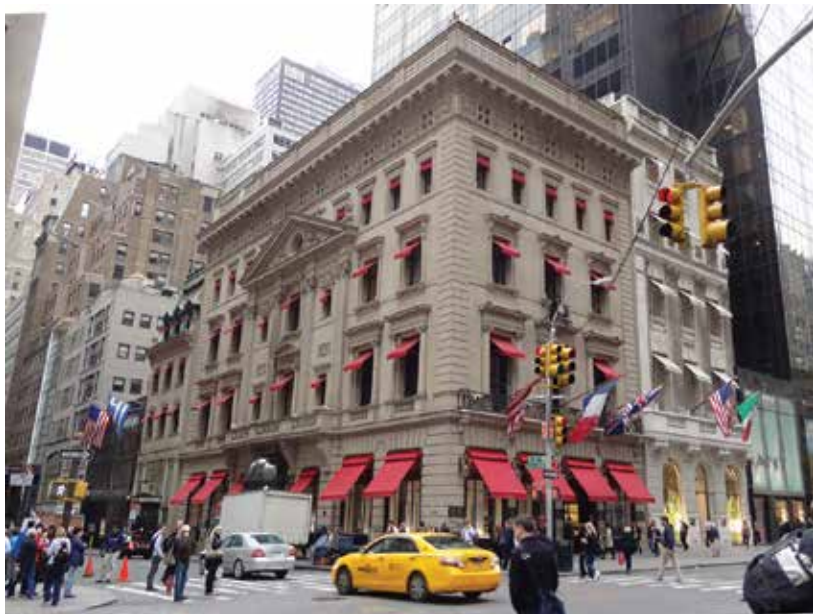
Cartier's flagship store, located at 653 5th Ave. in New York, was retrofitted in 2001 as part of a renovation.
